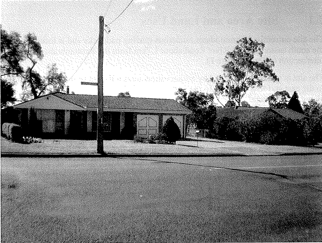
Photograph 1: A Typical Dual Garage House in Tahmoor
